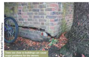
Trees too close to buildings can cause major problems for the owners
